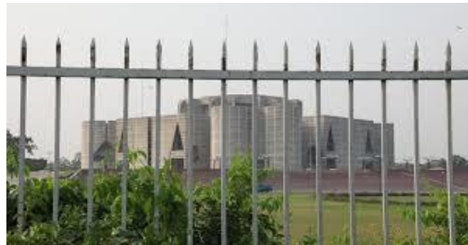
Boundary fence created for security of the complex, a breach to aesthetics and original concept of master architect Louis Kahn.
