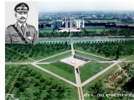
General Ziaur Rahman Mausoleum, 7 th president of Bangladesh; occupying his resting place which is violation to the original master plan
